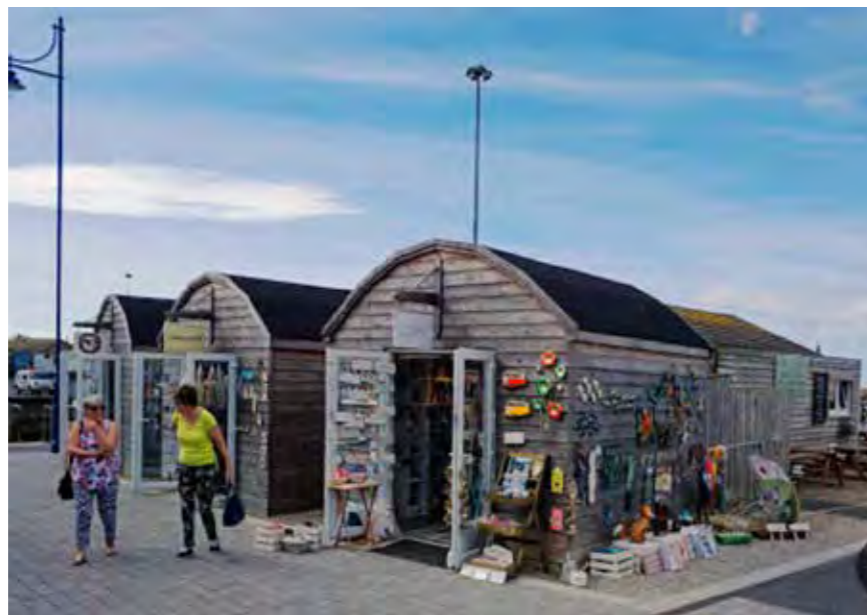
Gift shop Function: Doors open or closed Display: 3x internal shelves Spillout: Product display on external walls
