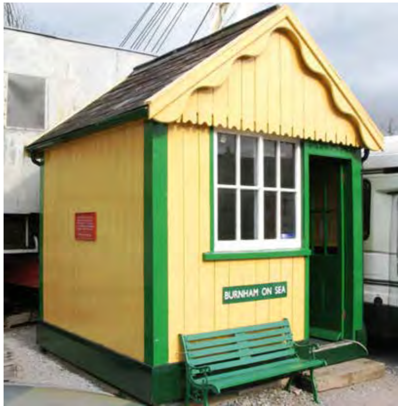
Burnham on sea signal box Size: 3x3m
